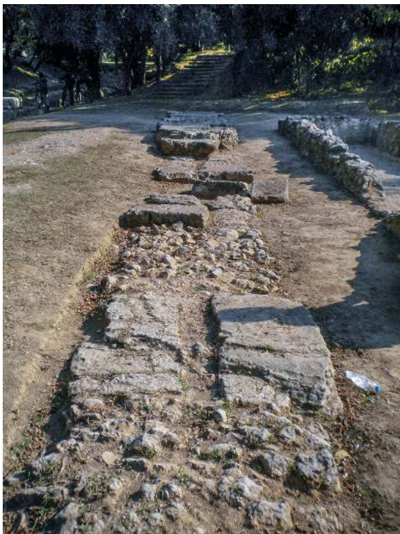
Fig. 4 Athens, Academy, so-called gymnasium: foundations of the northern portico, view from west.
