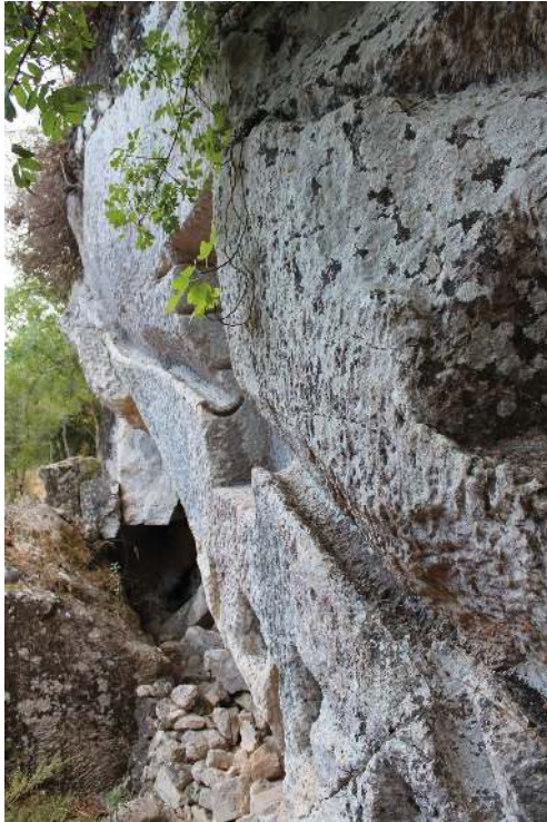
Fig. 11 Neaiton, 'gymnasion', channel in façade of caves 7 and 8, from N.
