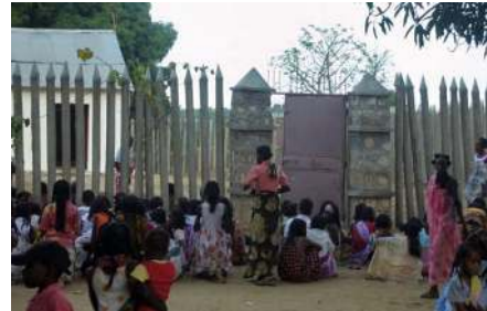
Fig. 8 The Doany Miarinarivo since 2000: the wooden palisade ( valamena ) has been replaced by concrete poles.
